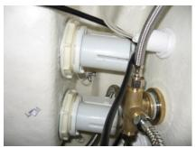
to the pump prior installation. Twist Pumps Counter Clockwise onto housing Plug in lock pin and power connectors
