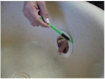
Step 4 Align the plastic O" ring adapter to cover completely Jet hole and use pencil to draw a circle. This will help you to line up the Jet before tighten the lock nut
