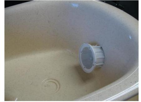
**Step 3** Disconnect Power & Remove. the defective Jet. Clean both sides of Jet Hole.
