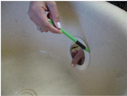
**Step 4** Align the plastic O” ring adapter to cover completely Jet hole and use pencil to draw a circle. This will help you to line up the Jet before tighten the lock nut
