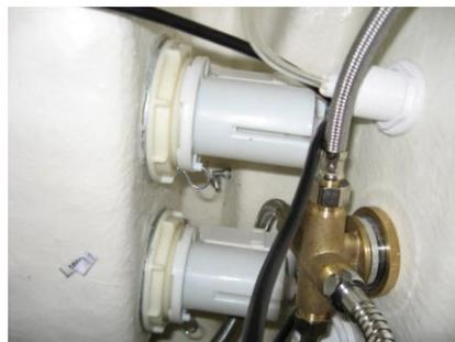
**Step 12.** Remember to return Black gasket to the pump prior installation. Twist Pumps Counter Clockwise onto housing Plug in lock pin and power connectors
