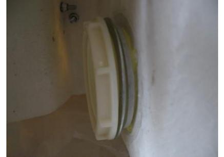
**Step 10** Slowly turn “clockwise” the lock nut . Avoid turning the housing.
