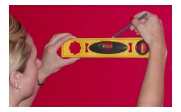
Take the horizontal mounting bracket piece (piece with tabs at top) and place it on the level line you drew. Mark the holes with a pencil and remove the bracket. Using a  $\frac{1}{4}$ " drill bit, drill the holes you just marked. Take the white plastic anchor and tap one into each drilled hole using a hammer. Make certain the anchor is flush with the wall.
