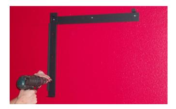
Line up the tabs on the horizontal mounting bracket with the two mounting cutouts located on the back of the backer. Lift the fireplace into position and make certain the tabs are locked into the mounting holes and the unit is seated securely on the wall. The tabs on the vertical bracket will sit under the backer.
