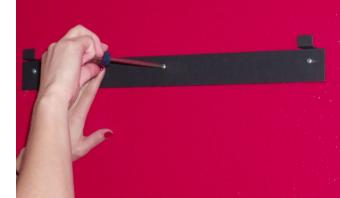
Place the horizontal bracket on the wall in line with the anchors and using the anchor screws secure and tighten the bracket to the wall. Hang the vertical brackets off each tab on the horizontal bracket. Using a level, level each side bracket and mark the holes.
