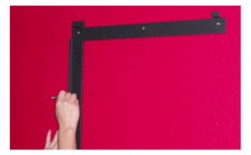
Remove the bracket and drill the newly marked holes. Tap into each hole one plastic wall anchor.
