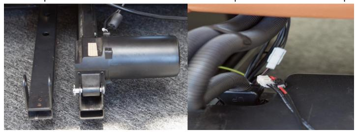
Install Bearing Block Guide using the 4 longer 1 ½" bolts and Allen wrench tool provided.
